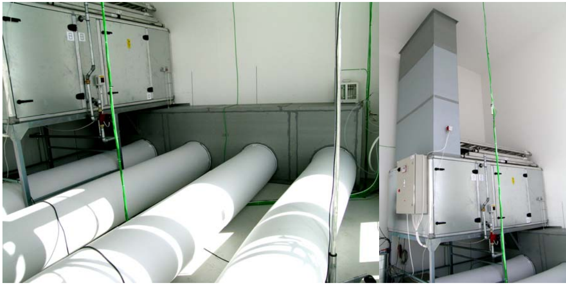
Figure 17. Ventilation recirculation system.
